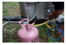
Connect the manifold refrigerant hose to the refrigerant supply tank. Verify the manifold's high & low side valves are closed before proceeding. Purge the air from the low side.
