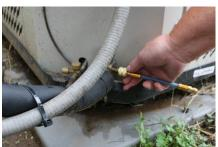
Turn the a/c system on, and verify the unit is running. Connect ProSeal XL4 Inject to the low-side service port of the system. (This is generally the large line.)
