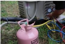
Connect the manifold refrigerant hose to the refrigerant supply tank. Verify the high and low side valves on the manifold are closed before proceeding. Purge the low pressure hose when connecting to the ProSeal XL4 Inject.
