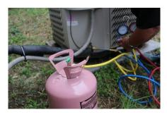
Connect the manifold refrigerant hose to the refrigerant supply tank. Verify the manifold high & low side valves on the manifold are closed before proceeding. Purge the air from the low side.
