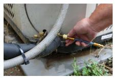
and verify the unit is running. Connect Air Enhancer Inject to the the system (This is generally the large line).
