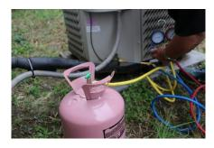
Connect the manifold refrigerant hose to the Verify the high & low side valves on the manifold are closed before proceeding. Purge the air from the low side.
